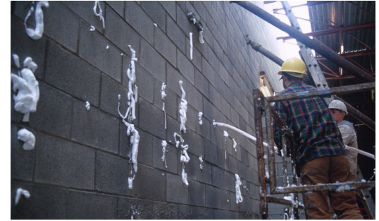
Fig. 4-4 Installation of self-expanding foam-in-place CMU core insulation
