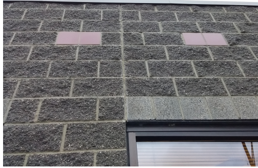
Fig. 4-5 Vertical CMU control joint
