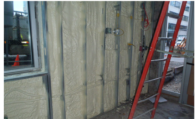
Fig. 5-4 Closed-cell spray foam insulation installed between steel studs
