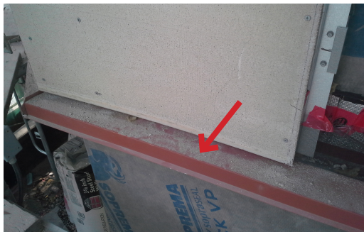
Fig. 6-10 Cross-cavity sheet-metal flashing shown below cement backer board
