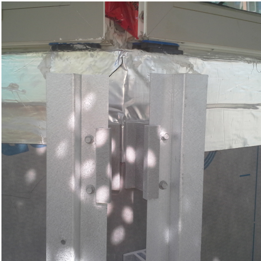
Fig. 6-11 Hot-dipped galvanized steel Z-girts attached to fiberglass cladding support clips
