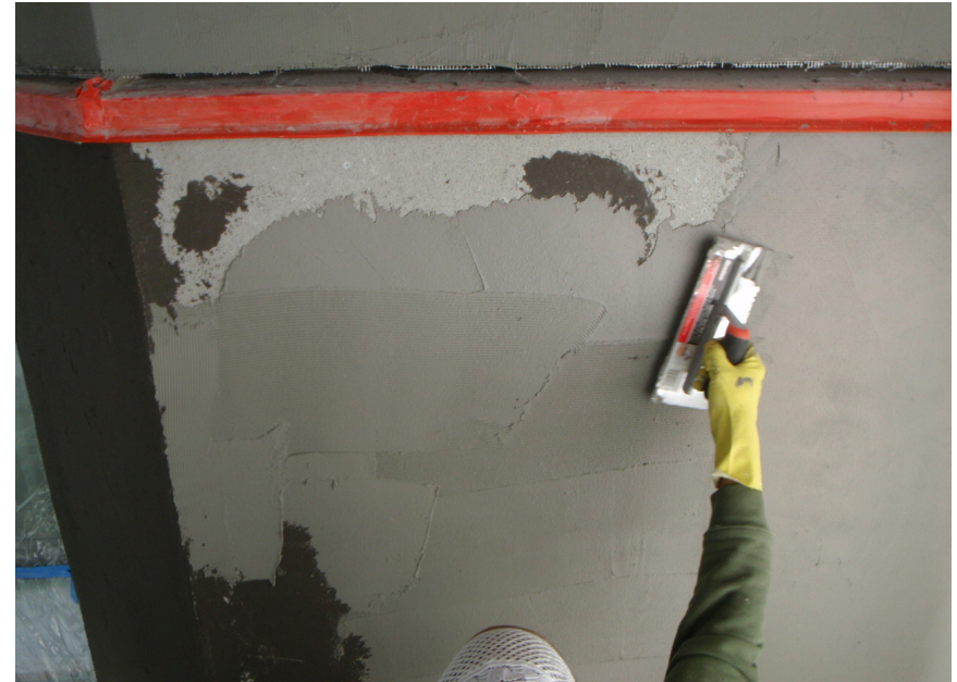
Fig. 6-13 Crack isolation membrane application over cement backer board. Cement board corners and fastener locations are treated prior to membrane application. A trowel-applied membrane is shown; membranes may also be fluid-applied.
