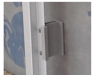
Fig. 6-5 Cladding support clip options modeled include intermittent Z-girt (top) and fiberglass standoff clip (bottom)
