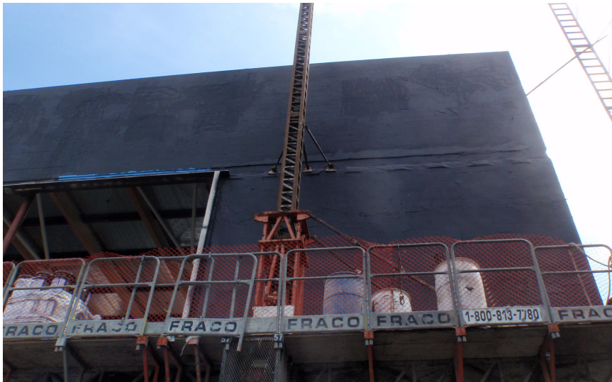
Fig. 6-4 Fluid-applied AB/WRB field membrane installed over CMU wall substrate
